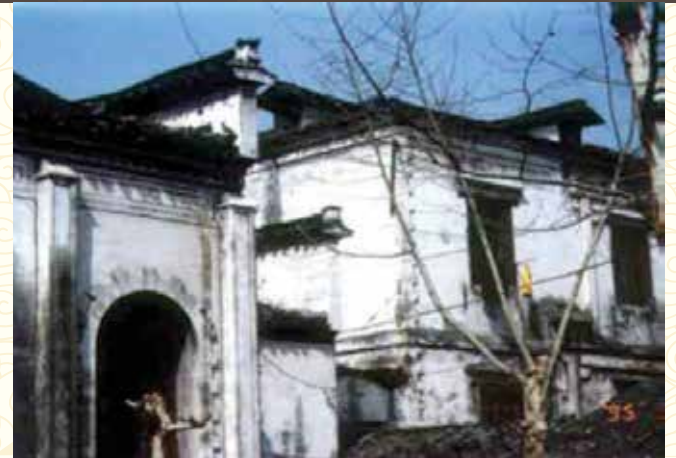
本會在歙縣的古老建築 Old Structures of the former Claretian Mission (She Xian) Estructura de la antigua misión Claretiana (She Xian) Struttura dell'antica missione Claretiana (She Xian)
